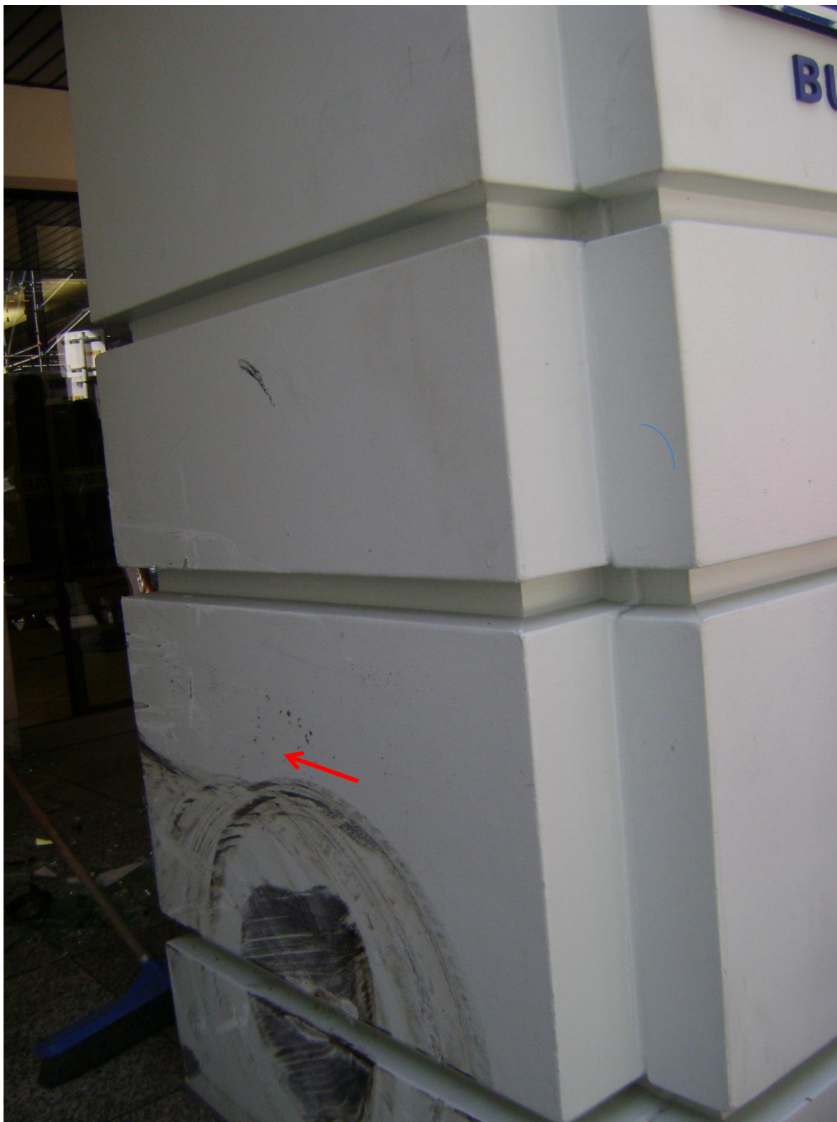
Fig 13 Circular scuff marks on pillar that appear to have been caused by rotating RH front tyre.
